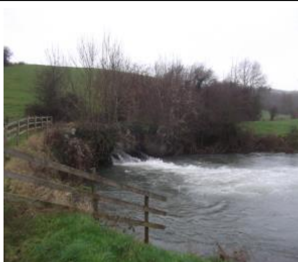
G: In-channel structures have lead to over-deepened channels and are an obstruction to fish passage.
